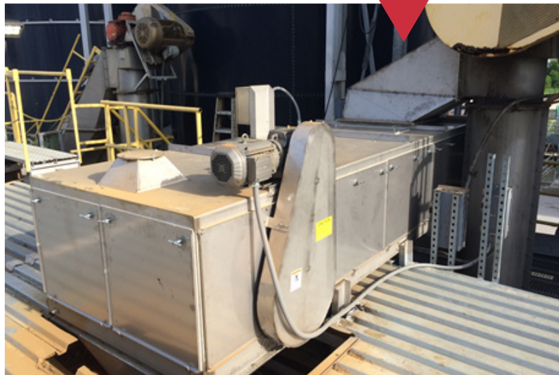
Thayer Weigh Belt in Place of Screw Conveyor
