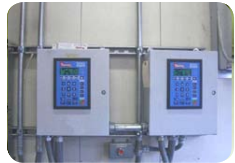
Series 5200 belt Scale Controller and Integrator used for "Master-Slave" ratio of Coal and Biomass
